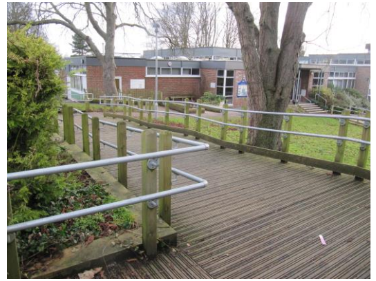
Pedestrian access ramps to Junior School
