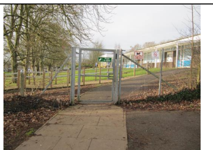
Approach from east gate to Infant School entrance
