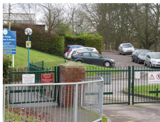
Entrance to staff car parks and pedestrian entrance. No safe footpath to Infant School reception. Nursery path leads off to the left.
