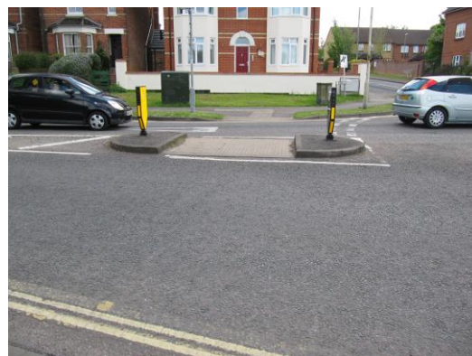
Pedestrian refuge on Worting Road from superstore car parks leading to Attwood Close
