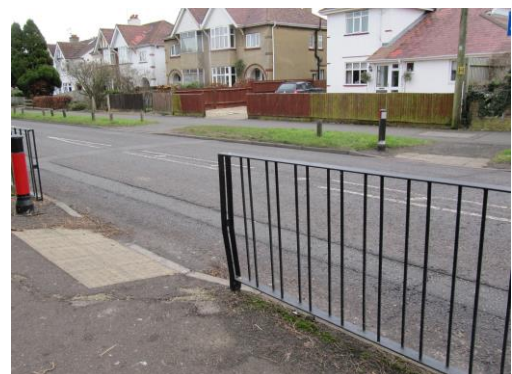
Dropped kerb crossing point on Winchester Road at the junction with King's Furlong Drive
