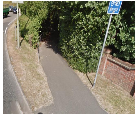
Entrance to the underpass from Winchester Rd near Portacre Rise - drainage recently upgraded
